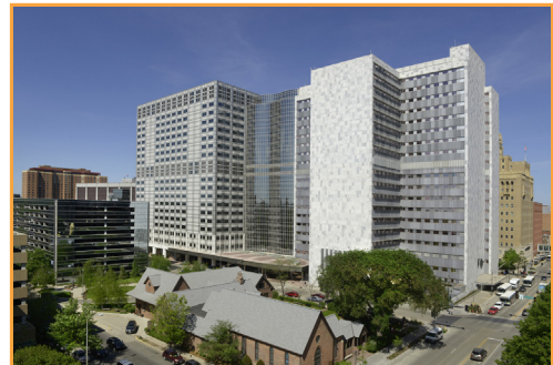
FIGURE 8. Most recently, the Department of Otorhinolaryngology moved from the Mayo Building to the Gonda Building on December 14, 2009. The new space includes 32 patient examination rooms, 13 double-walled sound booths for audiological testing, and 8 rooms dedicated to vestibular testing in addition to several procedure rooms, conference rooms, and separate office space. The Gonda Building can be seen between the Mayo Building on the right and Methodist Hospital on the left. Reproduced with permission of the W. Bruce Fye Center for the History of Medicine, Mayo Clinic, Rochester, Minnesota.
