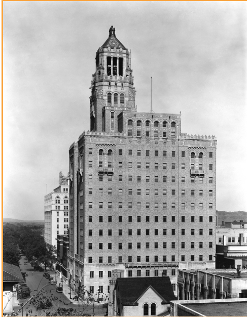
FIGURE 6. In 1929, all office work of the Section of Otolaryngology and Rhinology was transferred to Desk N-6 of the new Mayo Clinic building—now called the Plummer Building—and the entire corridor was assigned to the section. The space included 15 examination rooms and 1 room for vestibular testing in addition to separate staff office space. The new office was equipped with space for holding and storing medical records as well as a pneumatic tube system and vertical carrier for efficient transport of clinical records. At the time the Plummer Building was completed in 1928, it was the tallest building in Minnesota. Reproduced with permission of the W. Bruce Fye Center for the History of Medicine, Mayo Clinic, Rochester, Minnesota.
